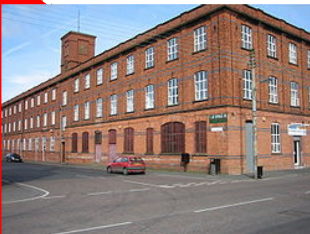
The former Johnston and Allen Linen factory on Victoria
